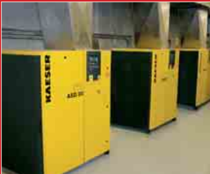
Top exhaust compressors facilitate energy-saving heat recovery without adding to system footprint.
