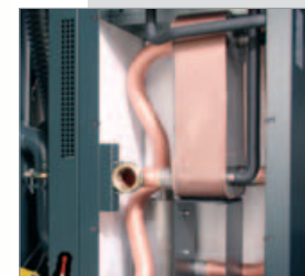
Thermal insulation omitted
