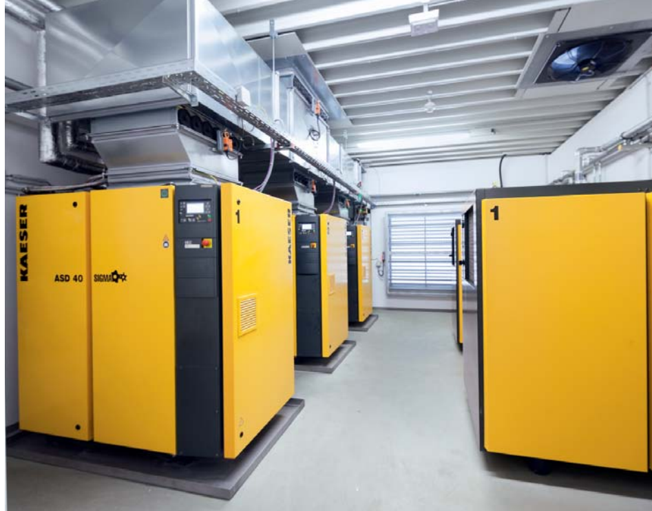
The 'Contracting' compressed air station at CP Autosport saves energy and money
