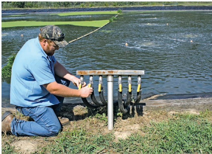
A city employee controls the airflow to each MARS unit in cell one by way of a stainless steel ball valve connected to a stainless steel air manifold.
