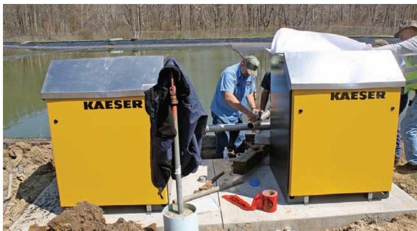
A city employee tightens the stainless steel header connecting the Kaeser blowers to the aeration units.
