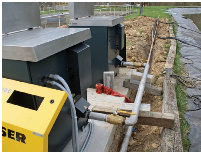
Two Kaeser CB 130C blowers and their header are tested for leaks before backfilling of the trench.
