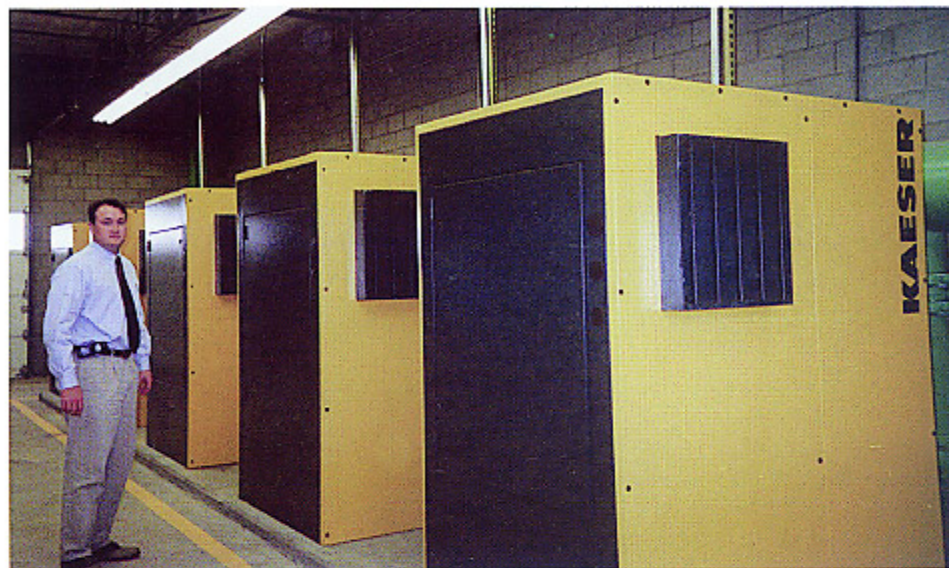
Steve Owen from PERC reviews the finalized installation of six FB 620 100 hp Omega-paks.
