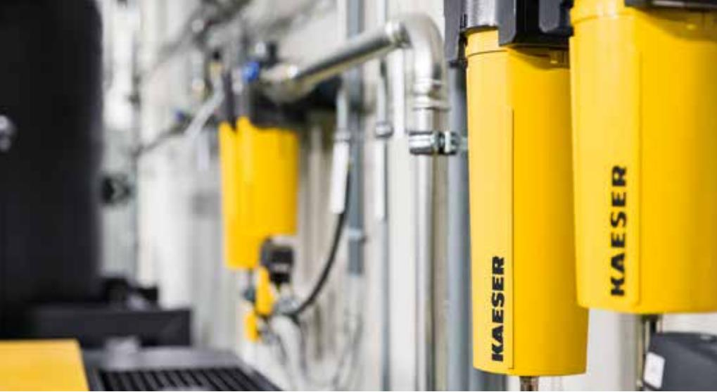
**Refrigeration dryers of types TL 1301 and ABT 25, active carbon absorbers, microfine upstream filters, downstream filters for achieving Particulate Class 1 (as per ISO 8573-1) and several other filter devices ensuring the high quality of the compressed air.**
