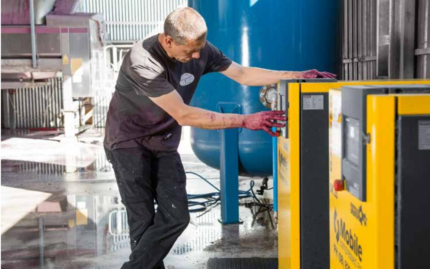
the requirements of the new plant, two KAESER SK 25 screw compressors and a 5,000 litre compressed air tank were purchased.
