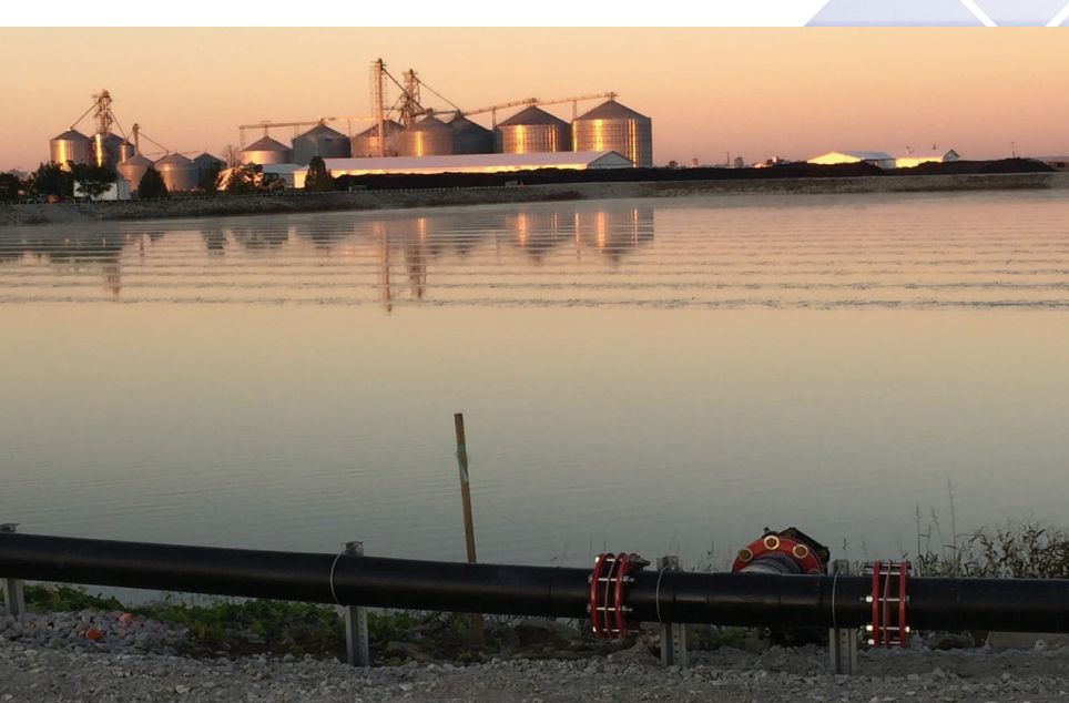
◀ ADS aeration lines producing zone of influence on the surface of the primary lagoon (left)
